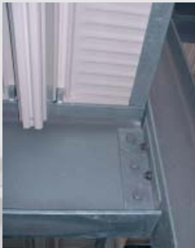
Positioning of trapezoidal profiles by using steel cleats.
