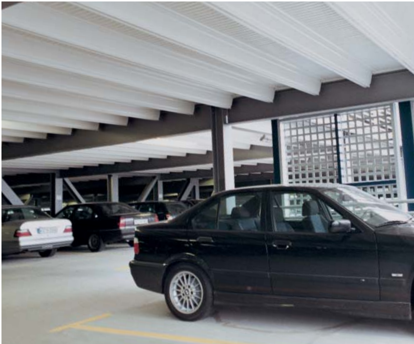
Parking deck in steel composite construction.
