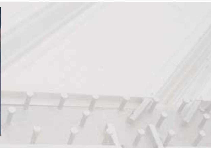
Positioning of trapezoidal profiles by using steel cleats.
